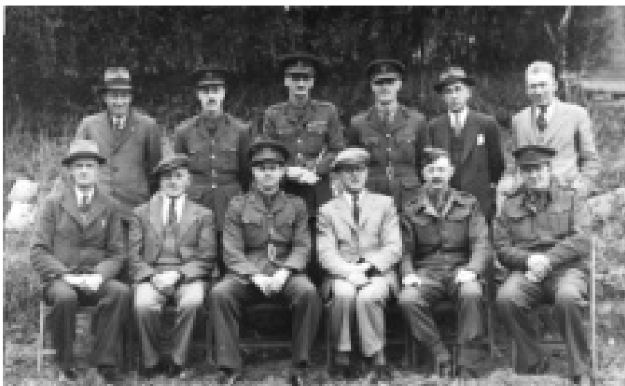
The Bailey Bridge Team. 1941.
