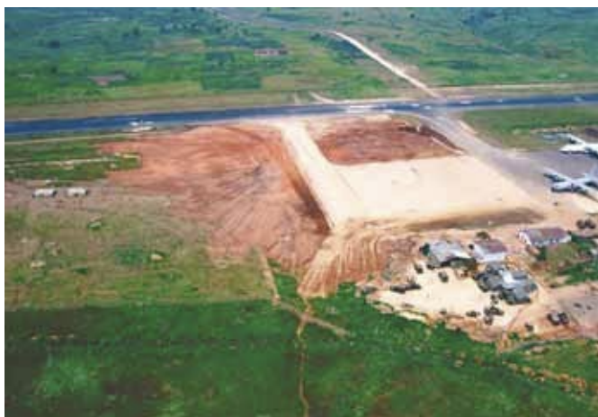
Aerial view from the North of finished apron
