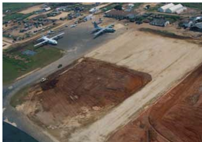
Aerial view from the South East of finished apron
